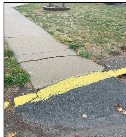
Existing/Current: Sidewalk Cut - Ben Allen Field House
