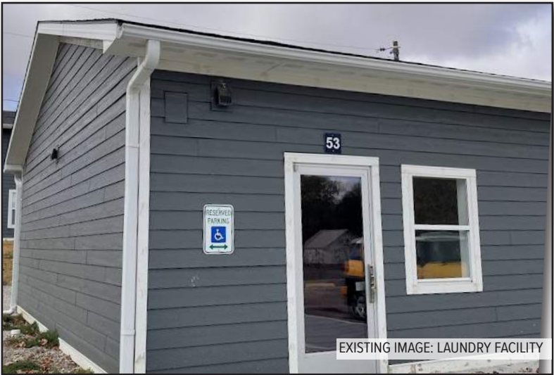
EXISTING FACILITY IMAGES:
