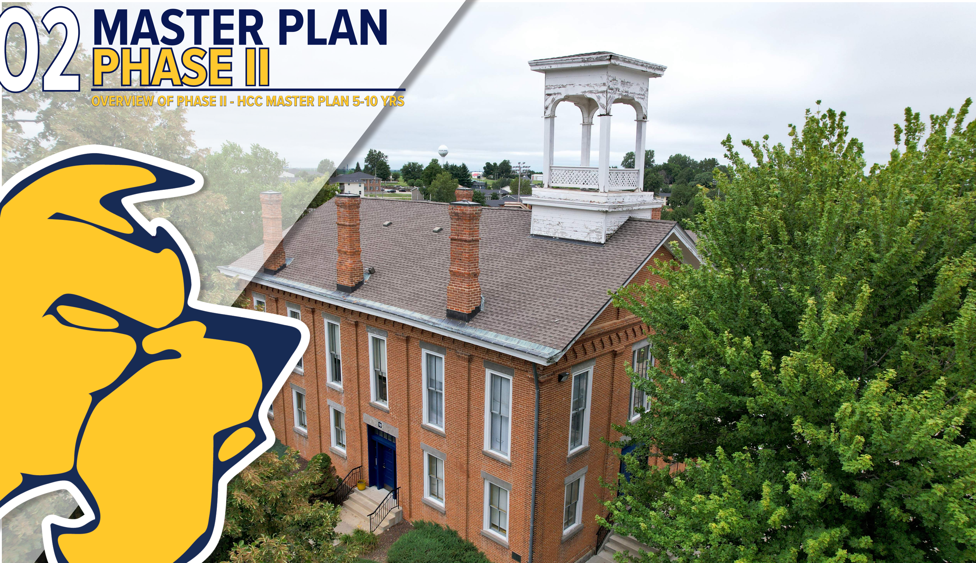
EXISTING IMAGE OF IRVIN HALL
