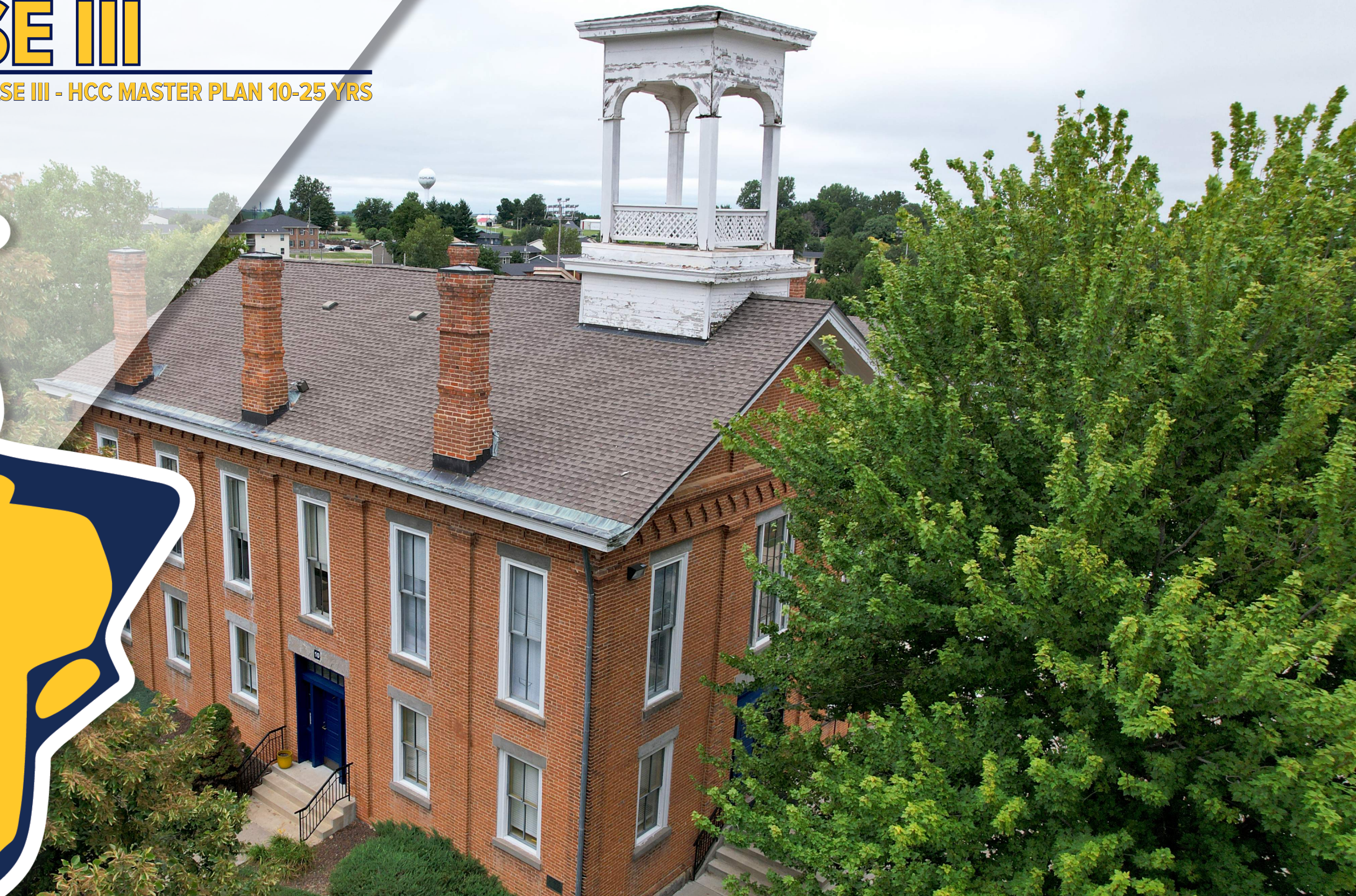
EXISTING IMAGE OF IRVIN HALL
