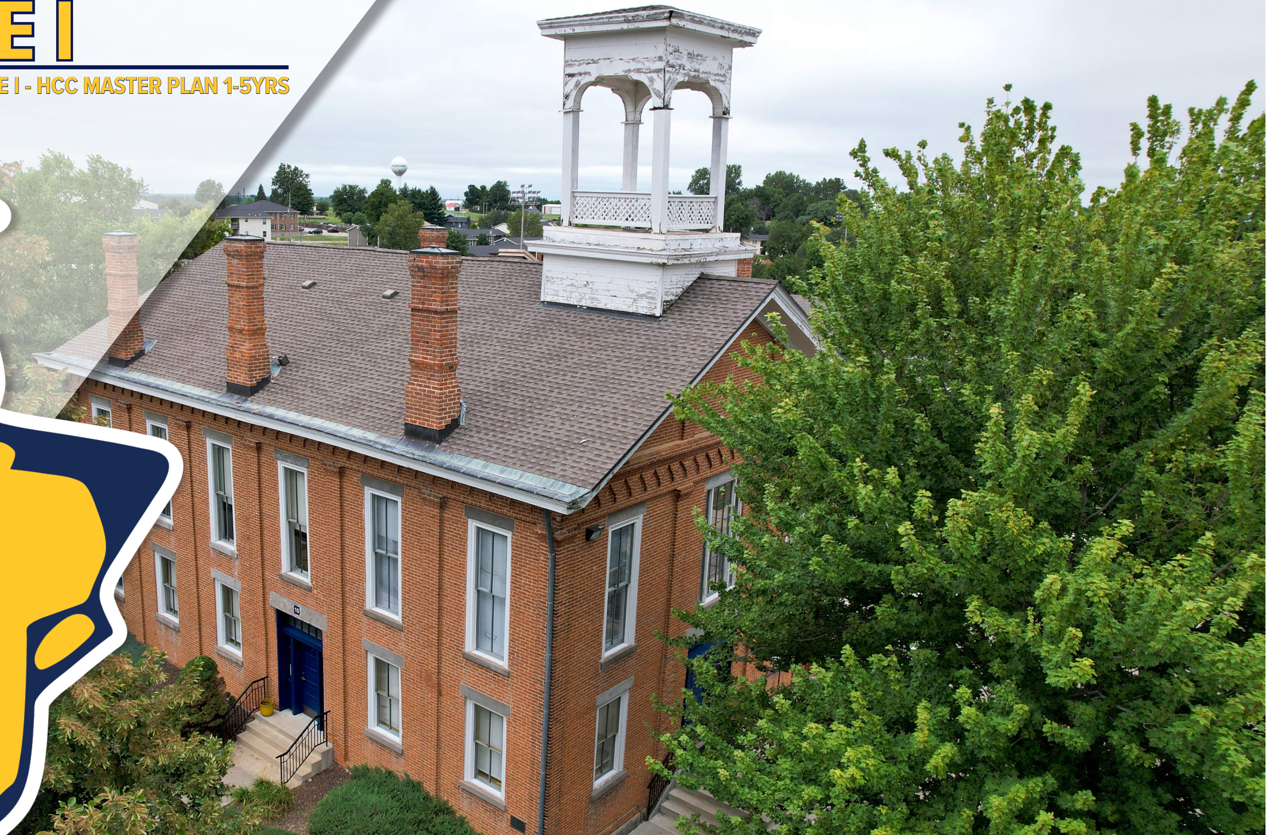
EXISTING IMAGE OF IRVIN HALL
