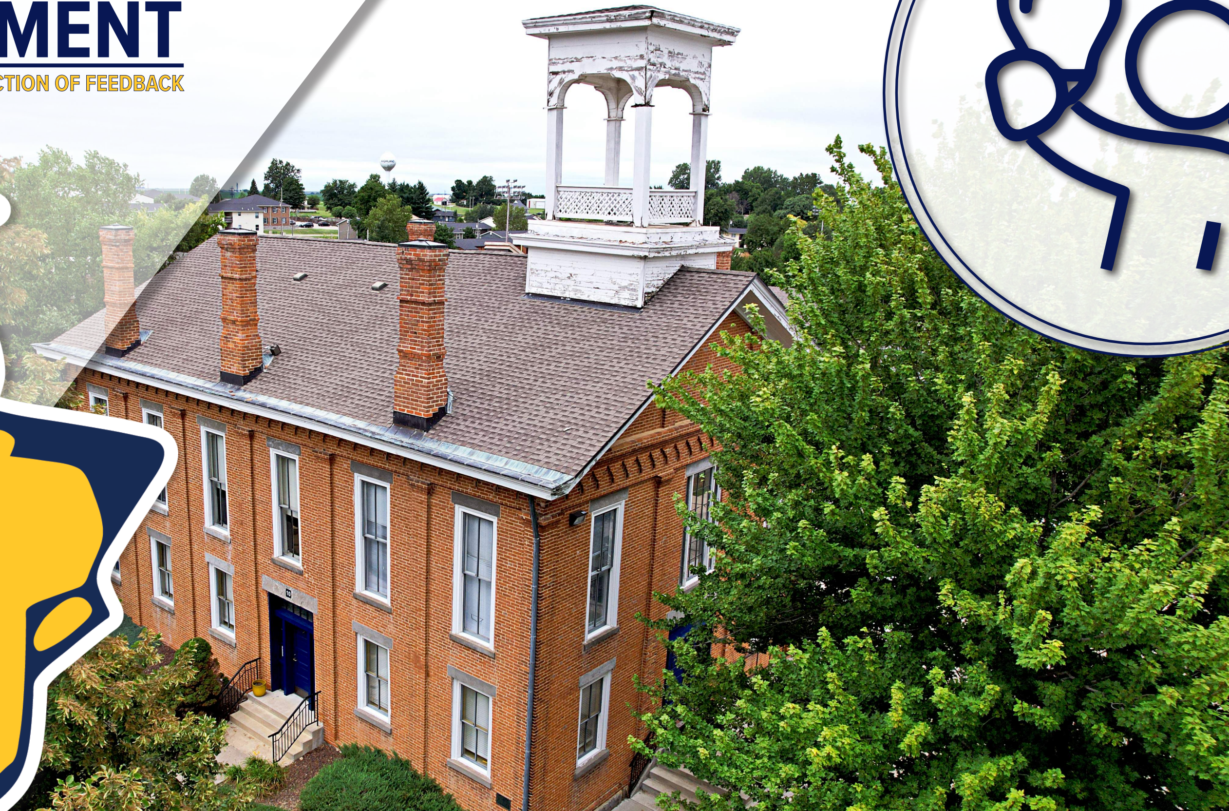
EXISTING IMAGE OF IRVIN HALL
