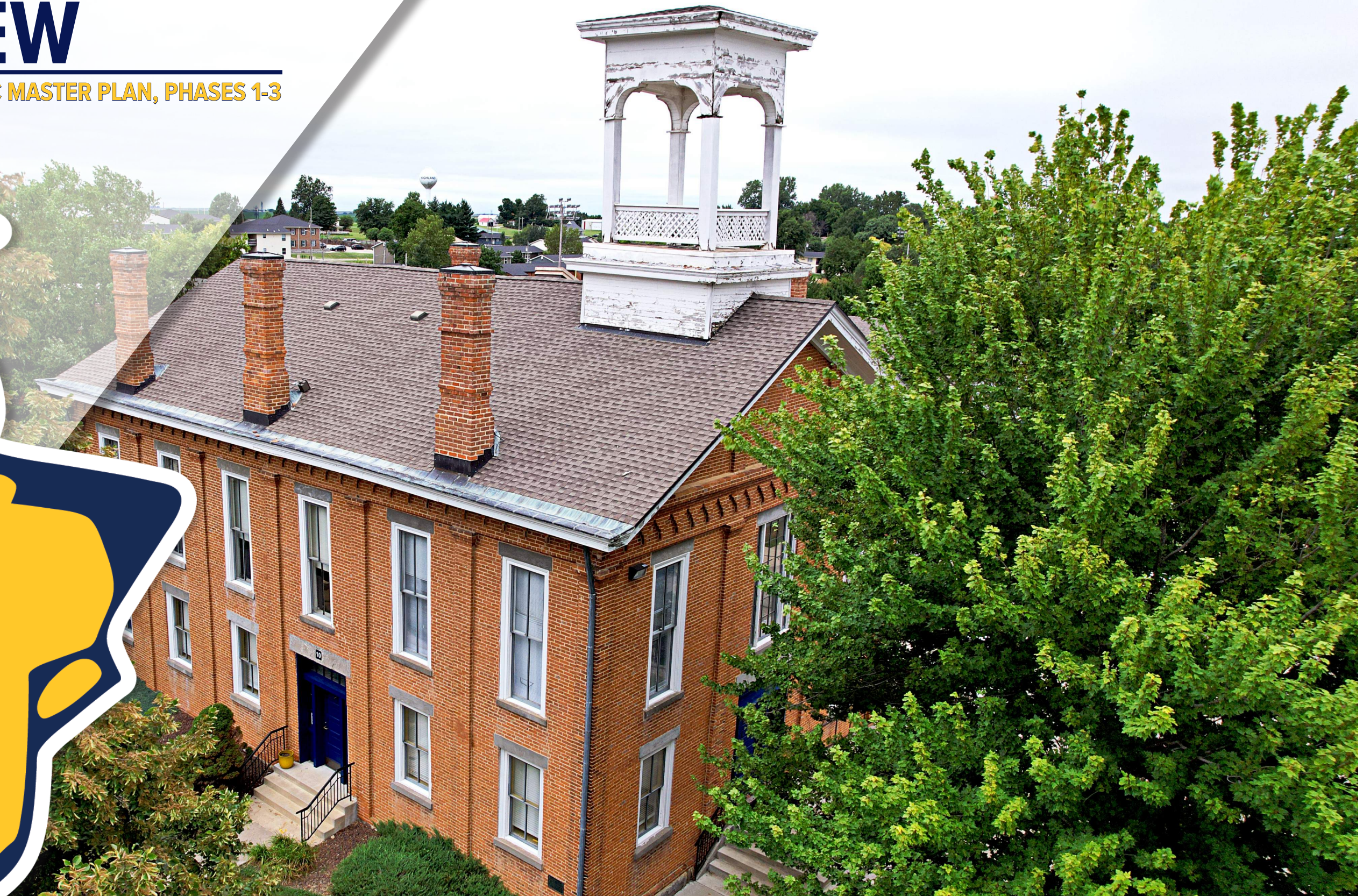
EXISTING IMAGE OF IRVIN HALL
