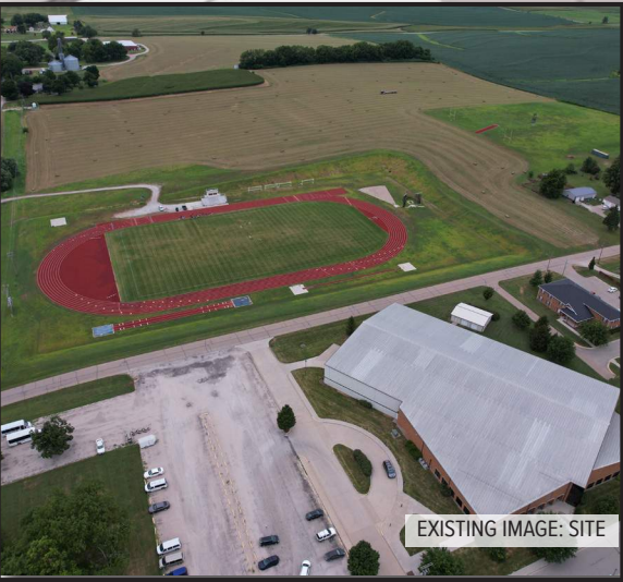
EXISTING FACILITY IMAGES:
