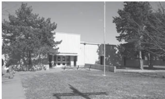
HCC at Perry Facility
